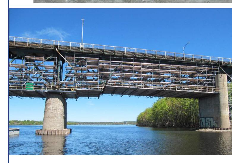
HI-LITE also provides a complete System Scaffolding solutions c/w standards, ledgers, ladders, clamps etc. Meeting all the CSA & DOT requirement for bridges.
